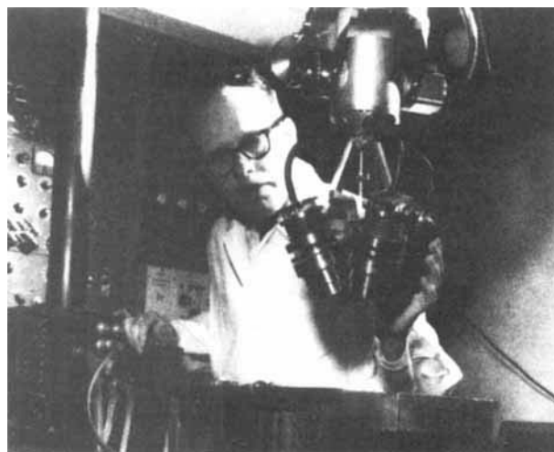
FIGURE 17. Dr. William Fry is shown with the transducer array he developed for producing pinpoint lesions in the central nervous system in animals and man. He is aiming four ultrasonic generators so that their beams are focused on a single point. (Reproduced with permission from University of Illinois Press, Urbana, IL.)
