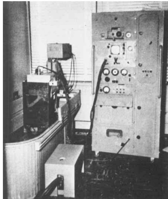
FIGURE 2. Cattle tank scanner developed by Dr. Douglas Howry and volunteers. The transducer carriage moves on the wooden rail along the side of the tank. (Reproduced with permission from Trans Am Clin Climatol Assoc 66:208, 1954.)
