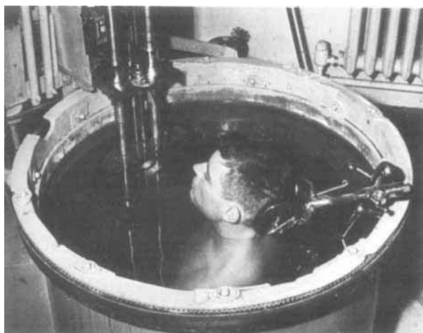
FIGURE 5. For scanning the neck, subject is immersed in the tank and a lead weight lies on his abdomen to prevent floating. The transducer carriage circles the neck. (Reproduced with permission from progress report to HEW, 1956.)
